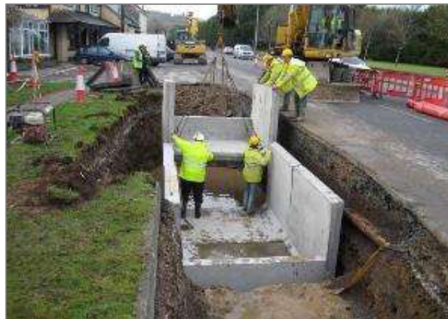
Figure 11: Typical joint bay under construction (pre-cast)
