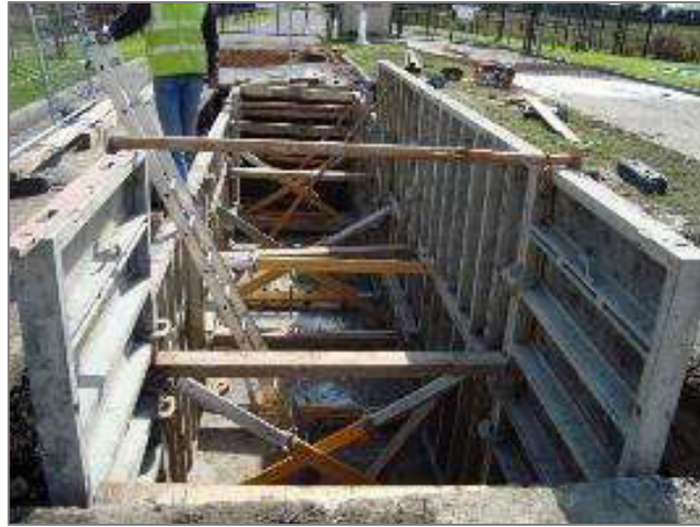
Figure 9: Typical joint bay under construction (in-situ)
