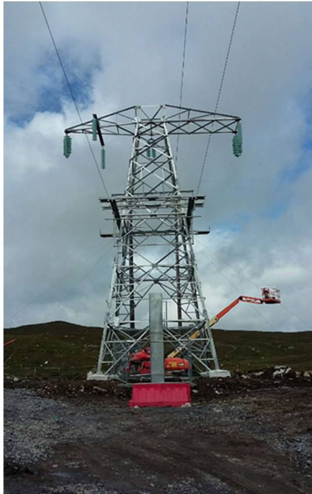
Figure 17: Completed Line/Cable Interface Mast
