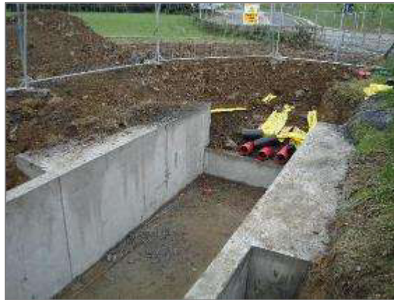
Figure 10: Completed joint bay prior to cable installation (in-situ)
