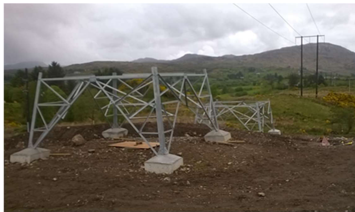
Figure 15: 110kV Interface Mast foundation complete
