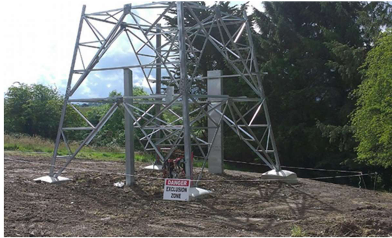
Figure 16: Base of Interface Mast structure backfilled
