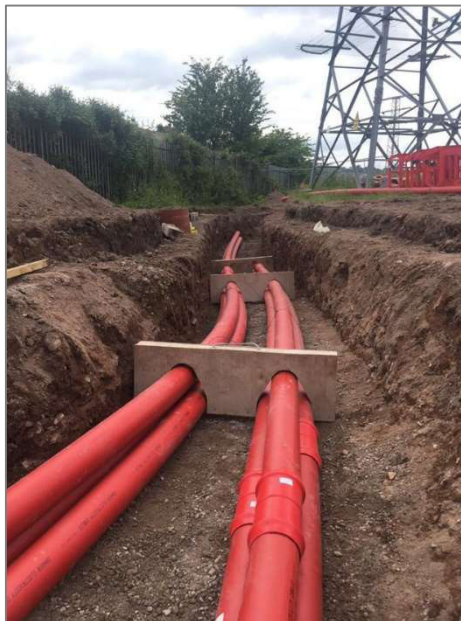
Figure 5: Double 110kV Underground Duct Installation
