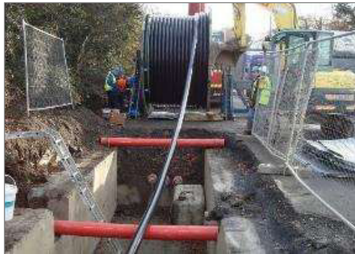
Figure 12: HV cable pulling procedure (Typical drum set-up)
